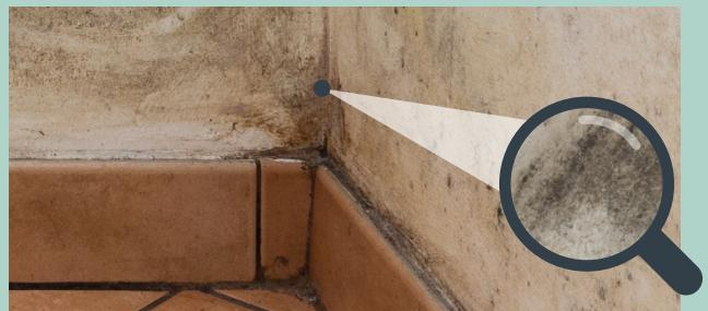
Groundwater rising up through floors and walls, usually due to damp proofing issues.
