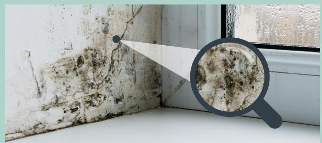
When warm air meets cold surfaces, it turns to water droplets. This is common around windows, in corners, and behind furniture.
